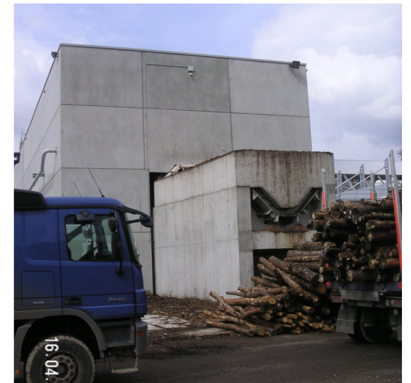
loading table to the bark stripper during operation
