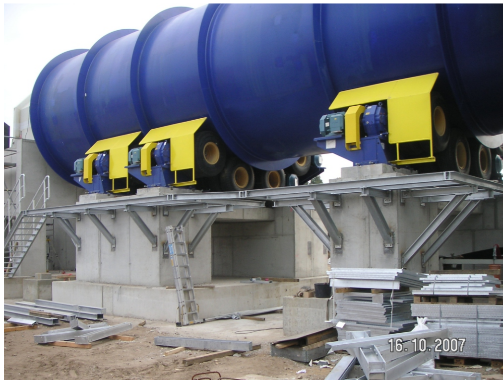
installation of the debarking drum
