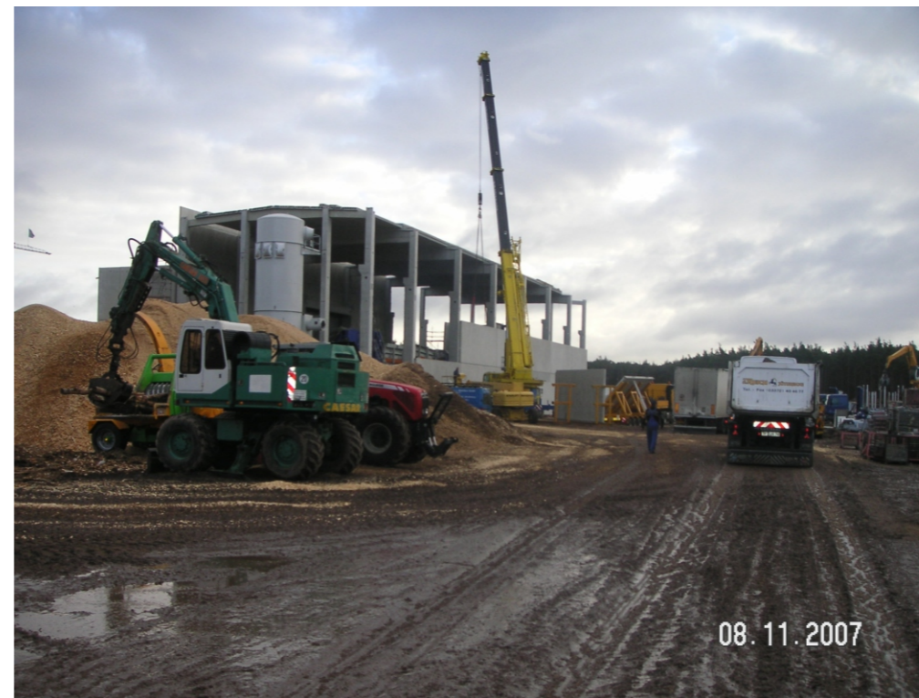
building during installation
