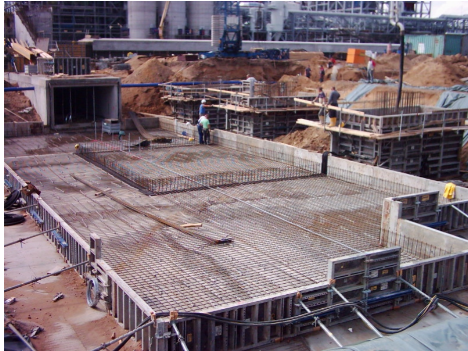
reinforcement base plate, in the background canal 2
