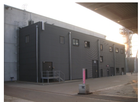
electric stock, control room
