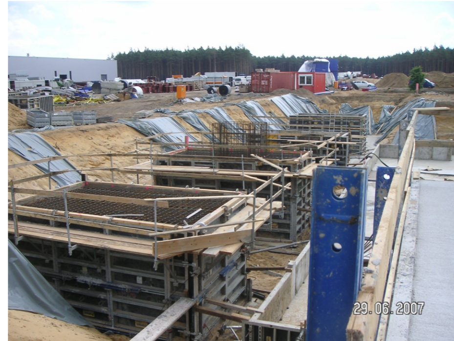
formwork column foundation
