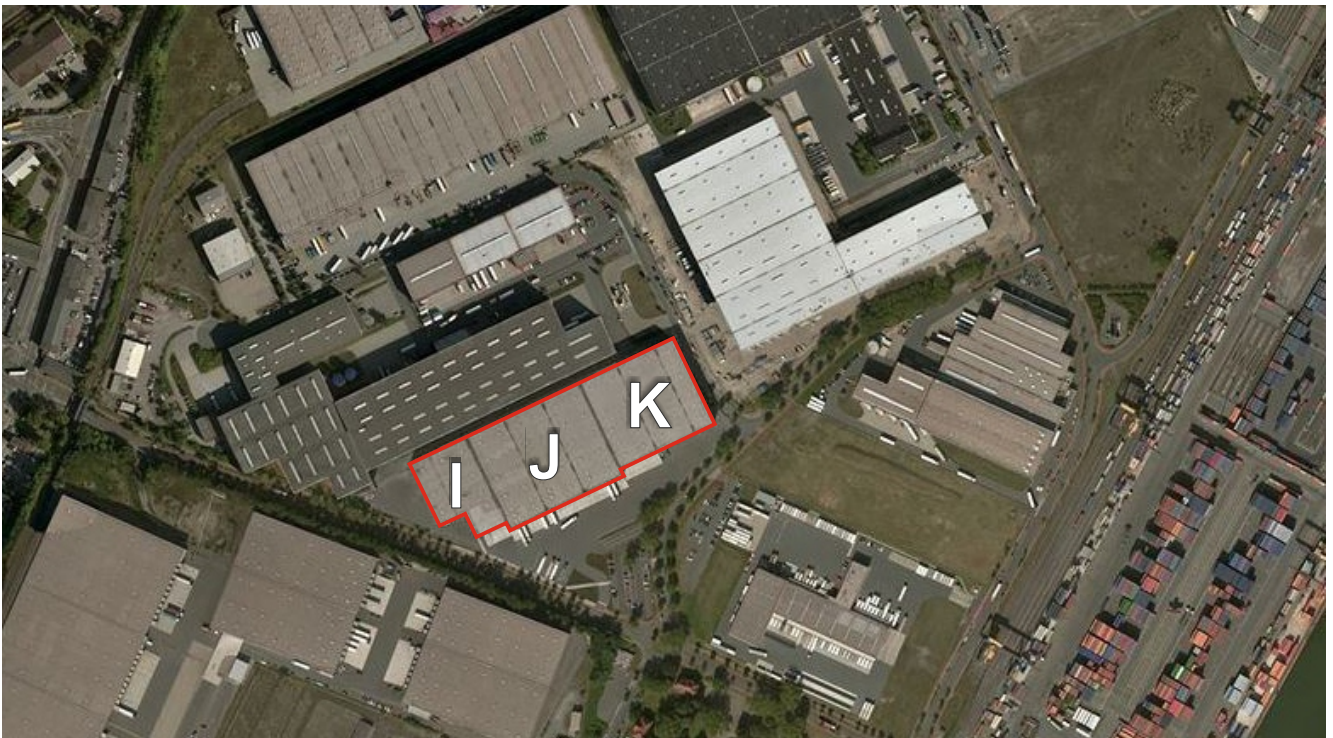
aerial photo Logport area
