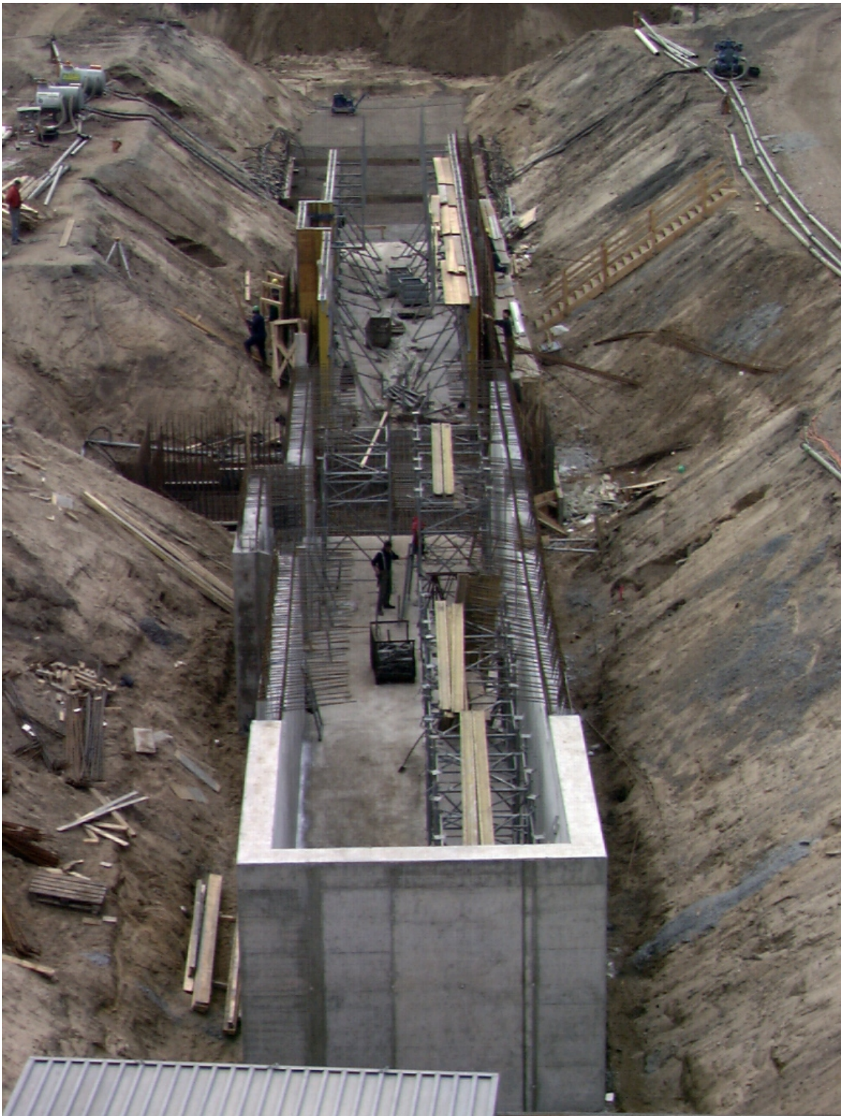
channel 1 (K1) while concrete work
