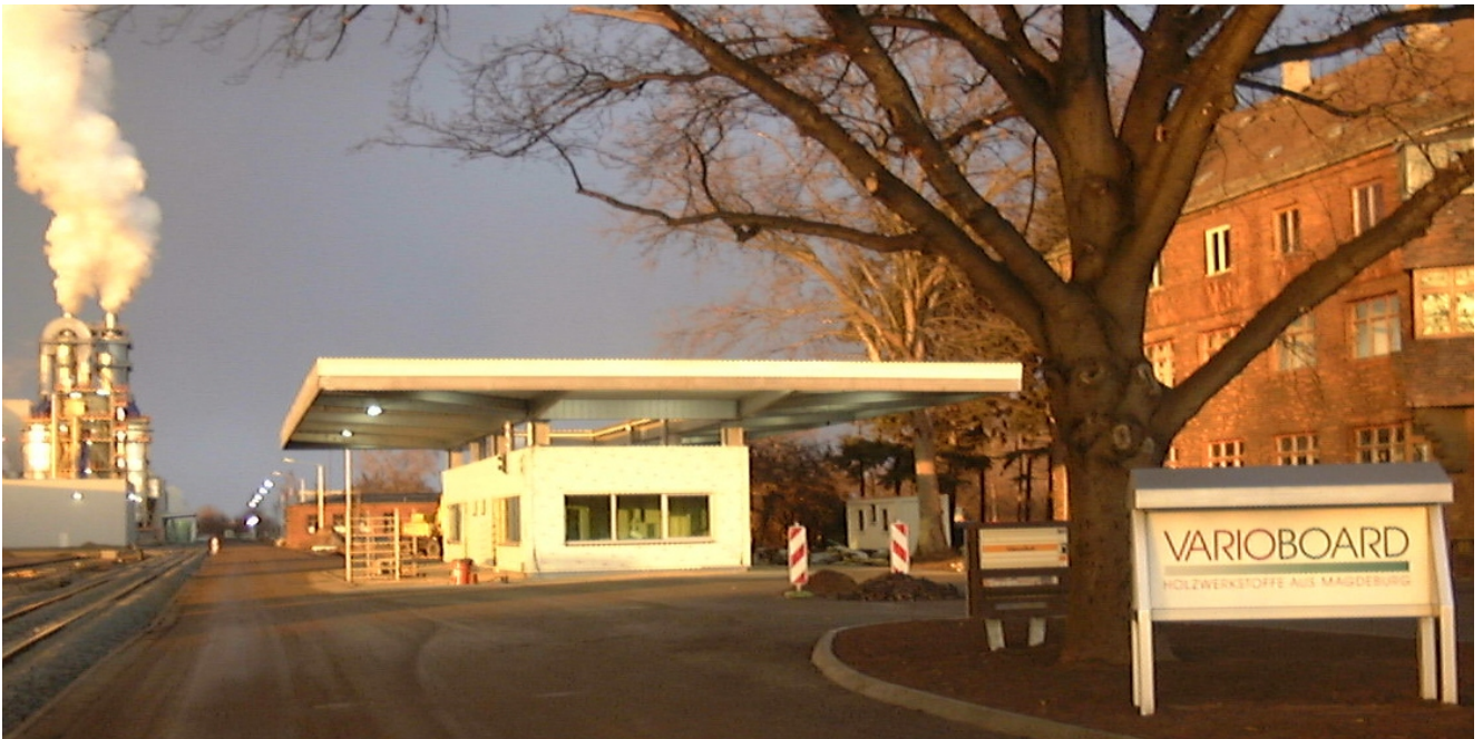
Gatehouse, Entry Varioboard area
