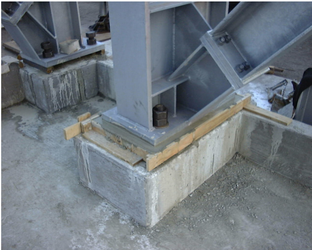
detail stanchion footing after construction
